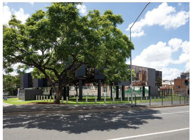
The ACCCE exterior view. (Source: RPS)
